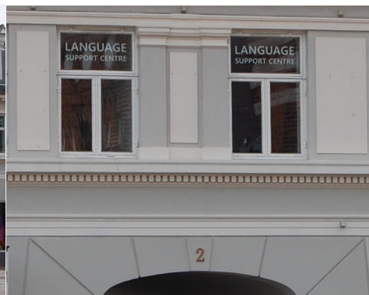
A detail over the entrance
